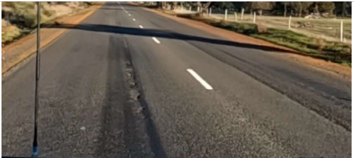
SLK 4.10 to SLK 4.20 – Flushing and potholes forming (WB Lane)
