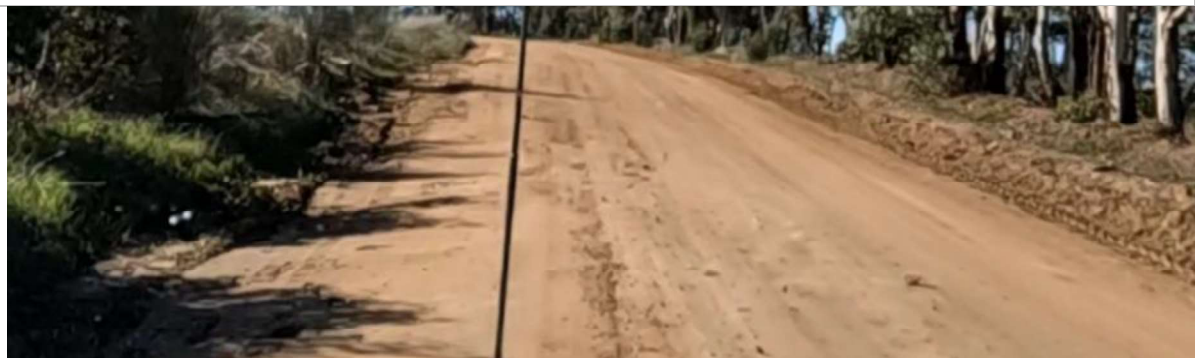
SLK 13.10 – Corrugations and uneven road surface resulted in poor rideability around bend
