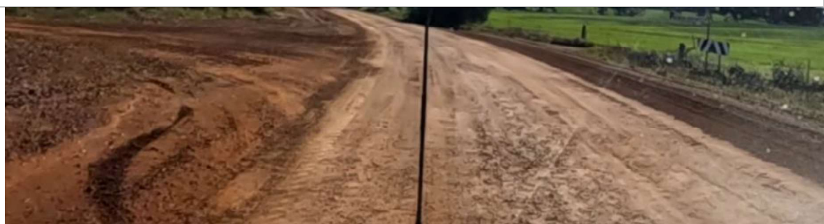
SLK 16.40 – Moderate corrugation, ravelling and potholes forming at Grahams Well Road intersection
