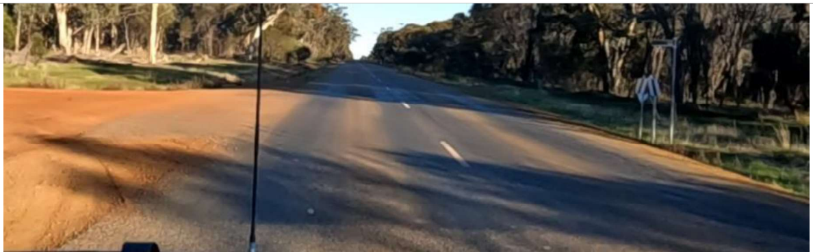
SLK 7.70 – Flushing near the intersection of Gittens Road
