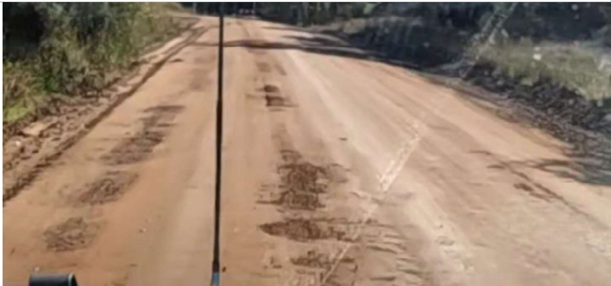
SLK 13.70 – Raveling and potholes forming
