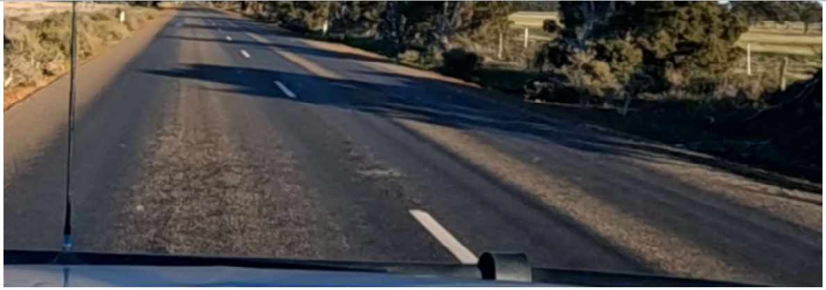
SLK 3.00 to SLK 3.30 – Flushing
