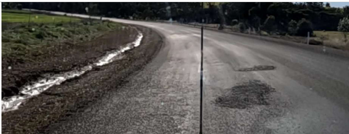
SLK 5.80 – Uneven road surface with minor raveling (NB)
