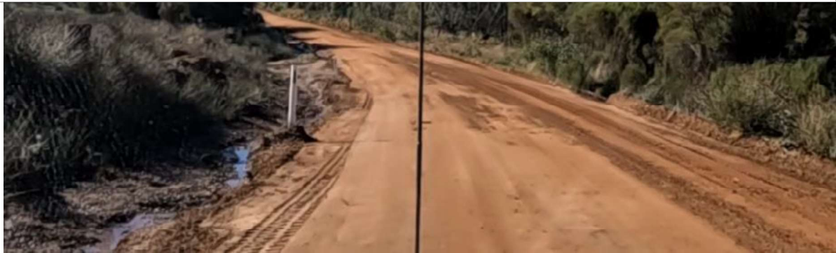
SLK 10.40 – Evidence of water ponding along the eastbound table drain
