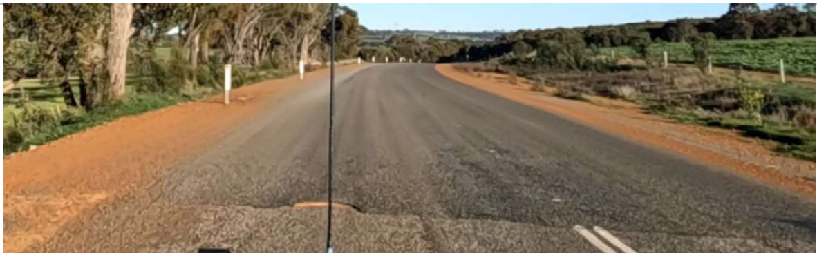
SLK 26.30 – Pothole forming at change of seal, No Linemarking
