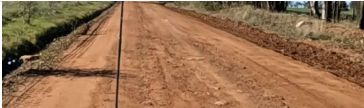
SLK 12.60 to SLK 12.80 – Moderate corrugation, rutting and raveling with potholes forming
