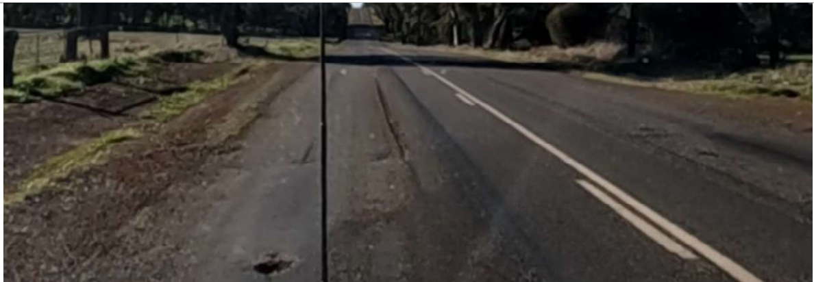
SLK 10.50 – Pavement seal patch failing with pothole and longitudinal crack (EB Lane)
