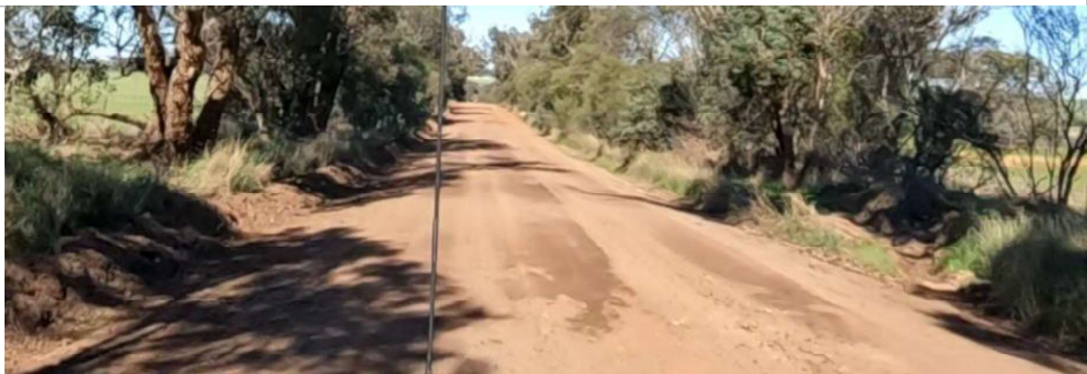
SLK 14.2 – Potholes, rutting and base course exposure
