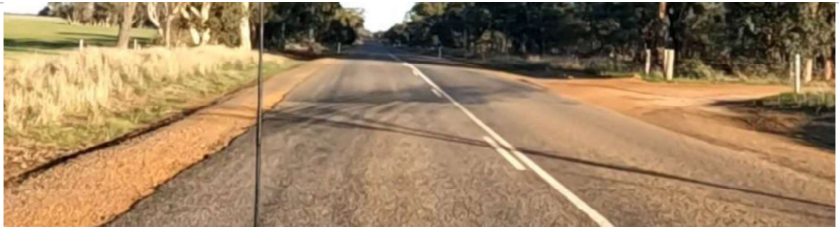
SLK 5.90 – Minor edge break and flushing near the crossover
