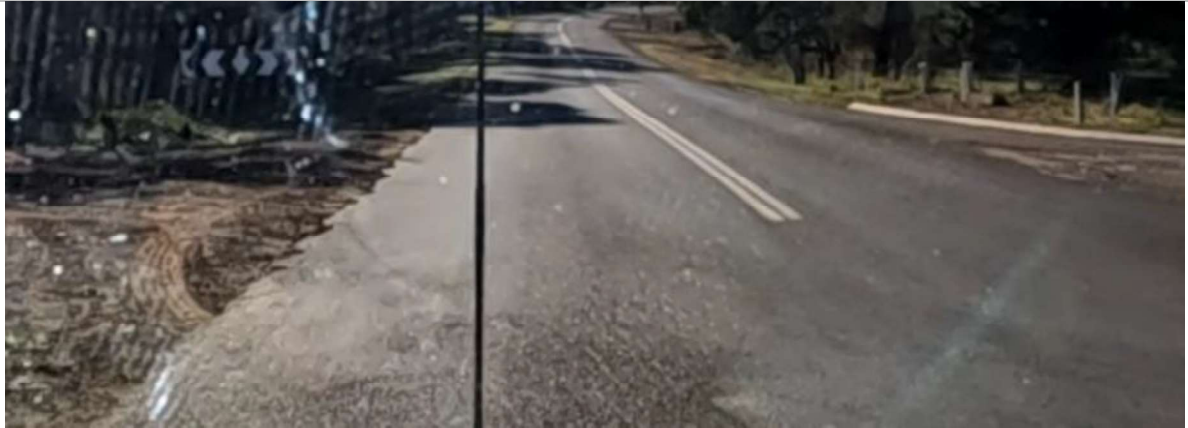
SLK 0.80 – Mild edge break (EB Direction)
