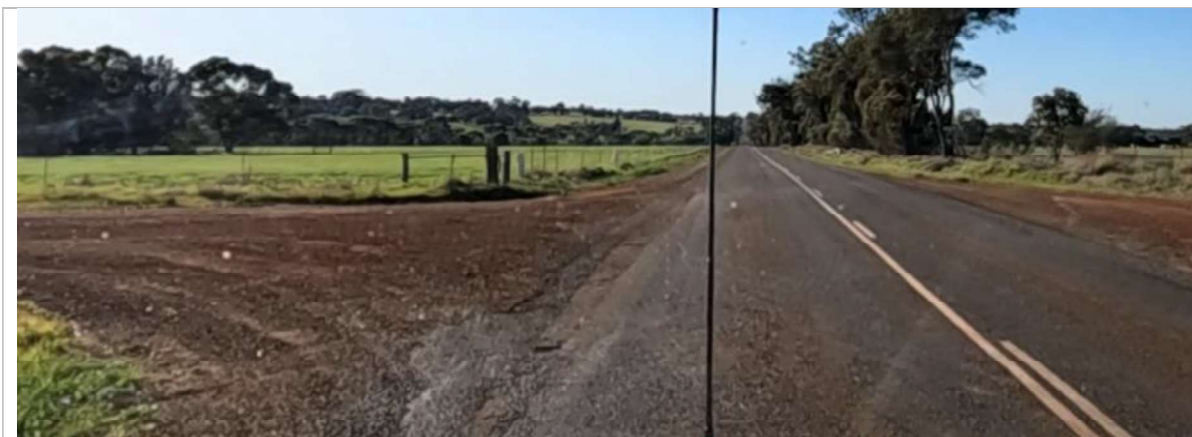
SLK 12.80 – Edge break and ravelling at Pindellup Road intersection
