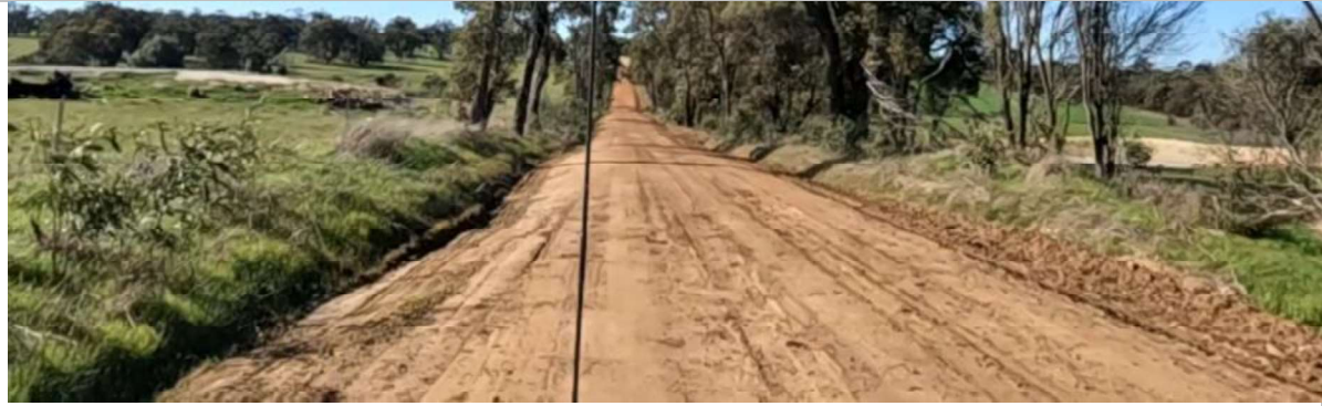
SLK 12.20 – Moderate corrugation, uneven road surface resulting in poor rideability
