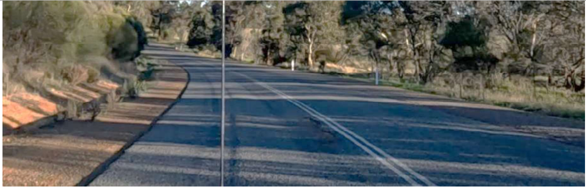
SLK 24.20 – Potholes near the centre line
