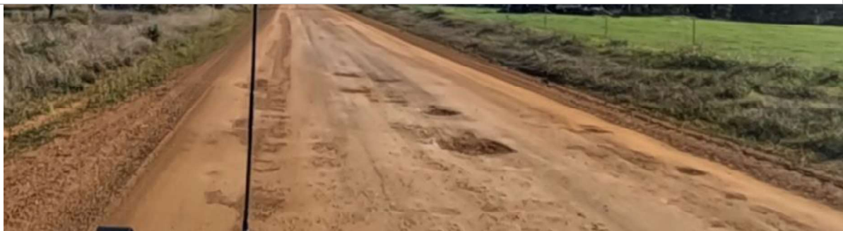
SLK 12.60 – Moderate corrugations with large potholes
