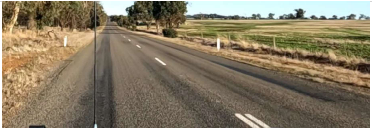
SLK 17.50 – Minor flushing
