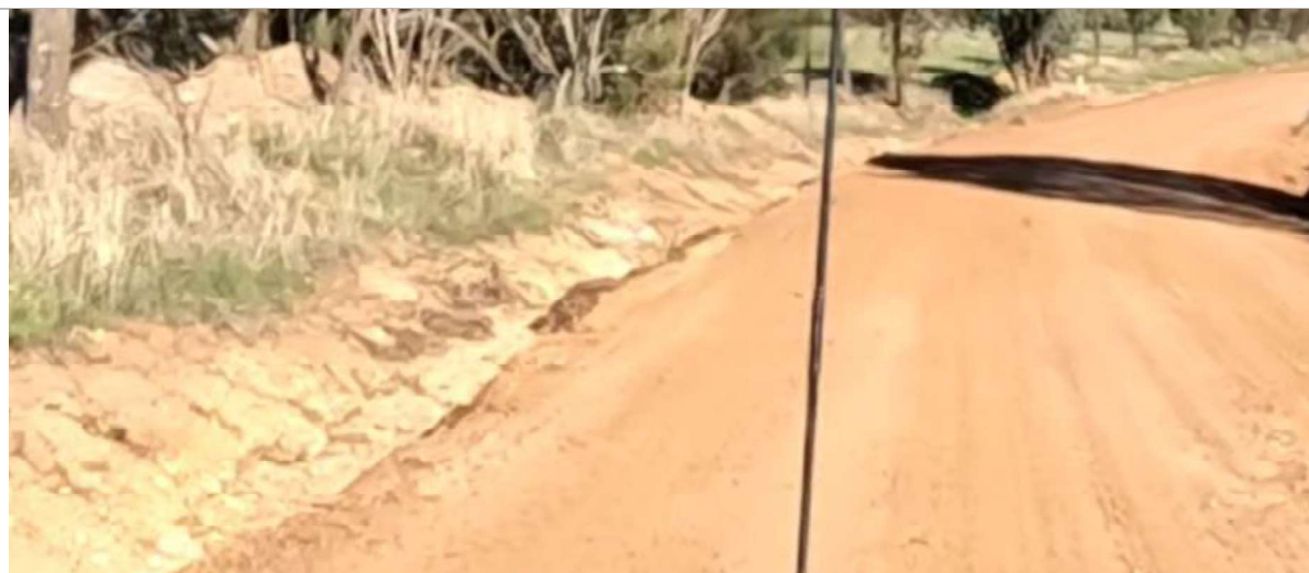
SLK 9.40 to SLK 9.60 – Drainage with large drop-off on the edge of carriageway (WB)
