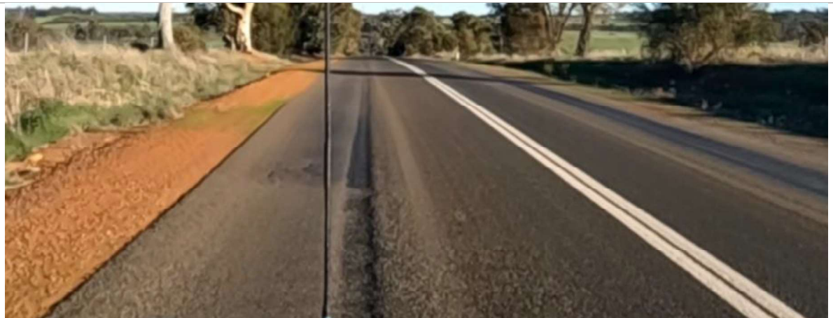
SLK 19.00 to SLK 20.00 – Minor ravelling and rutting along seal joint (WB)
