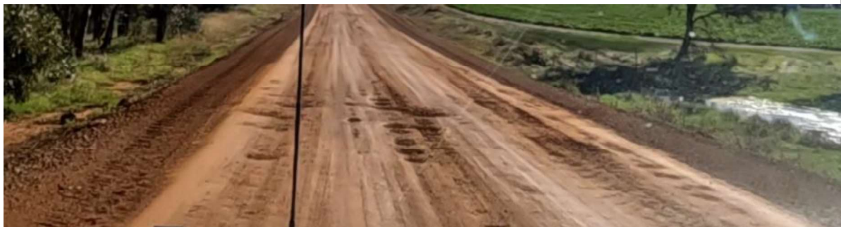
SLK 17.20 – Potholes near culvert
