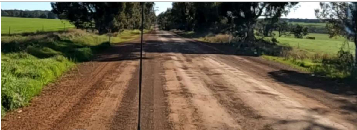
SLK 8.50 – Moderate corrugation and potholes
