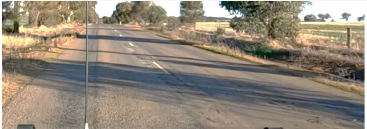
SLK 17.90 – Ravelling and potholes forming near the centre line
