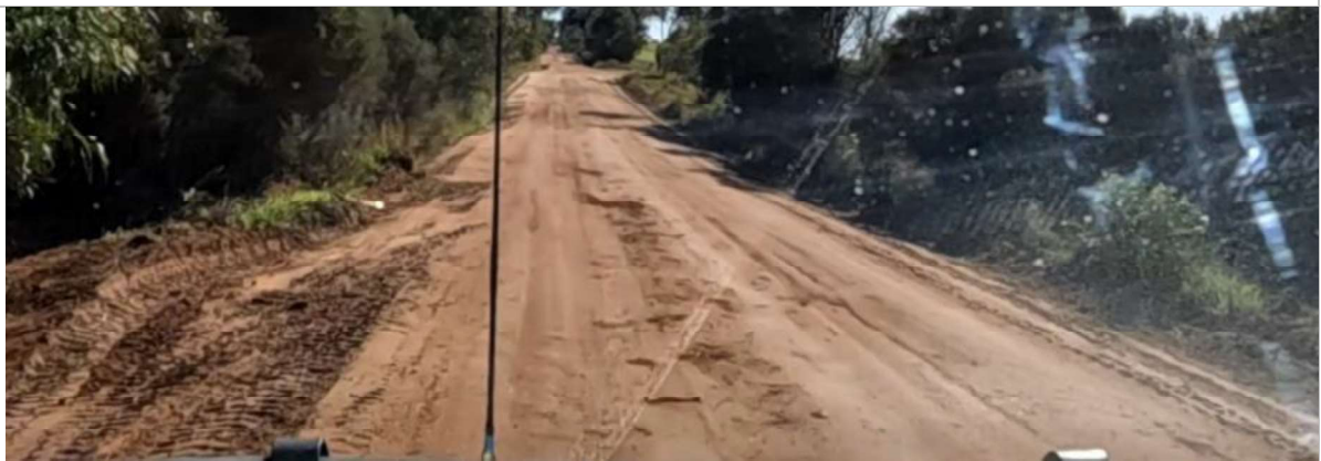
SLK 15.80 – Rutting and potholes forming
