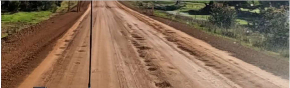
SLK 16.80 to SLK 17.00 – Severe potholes near Ngopitchup Road intersection
