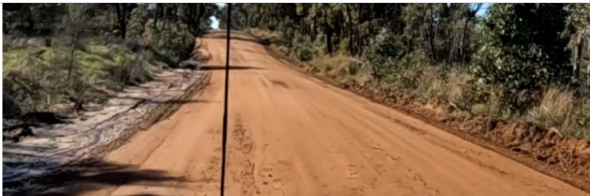
SLK 10.50 – Effective road width narrowed due to table drains around the bend (~4.5m)
