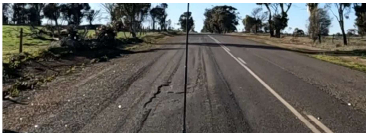
SLK 11.40 – Pavement Seal Failing with cracks and base course exposure (EB Lane)
