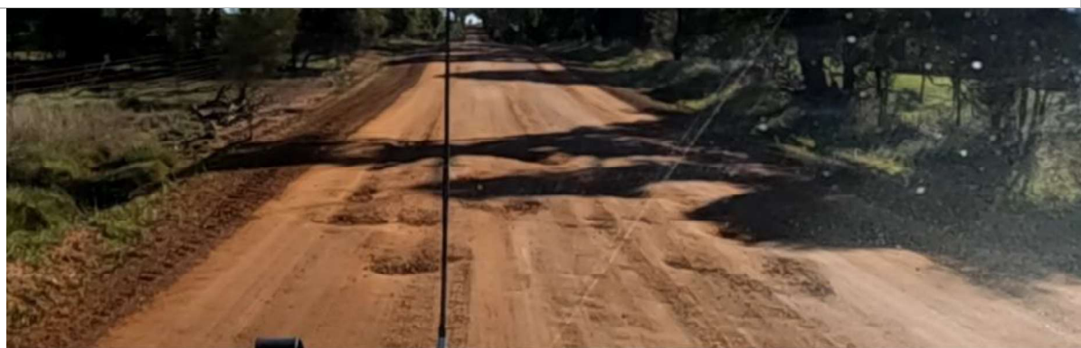
SLK14.80 – Moderate corrugations with potholes
