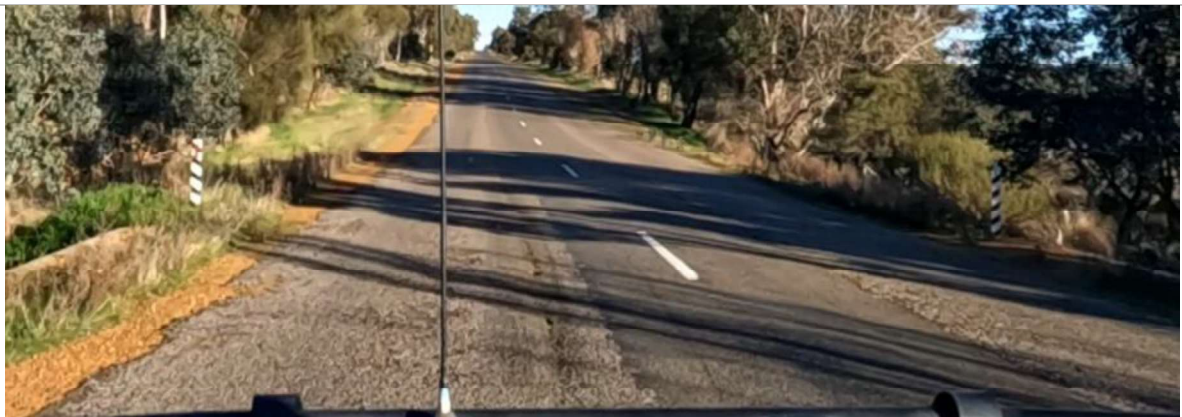
SLK25.00 – Minor edge break and potholes forming (WB)
