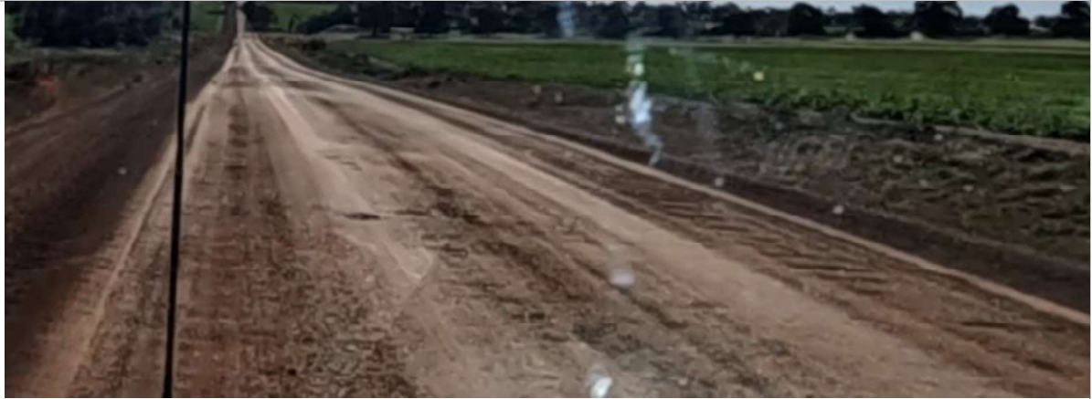
SLK 17.90 to 18.10 – Moderate corrugation, ravelling and potholes forming
