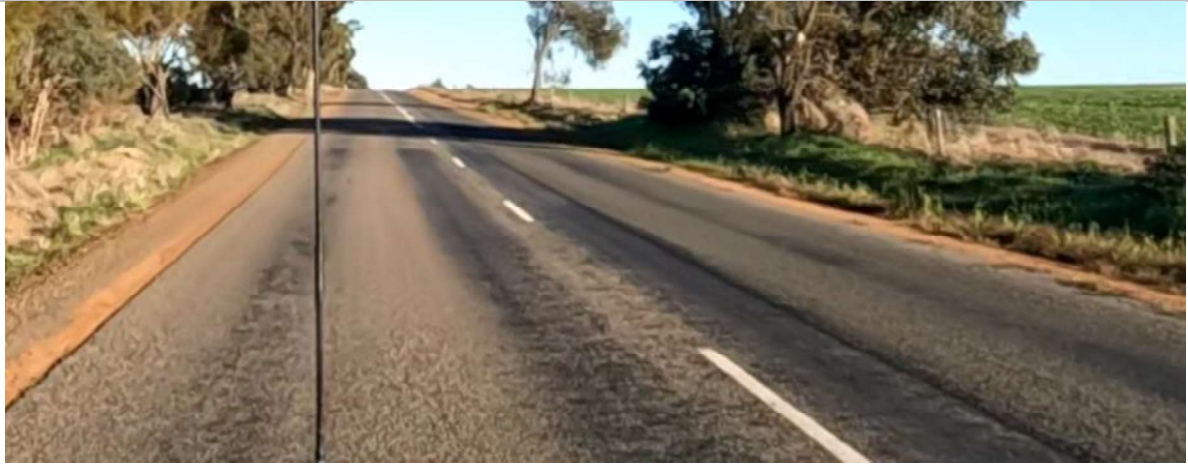
SLK 9.50 – Minor Flushing
