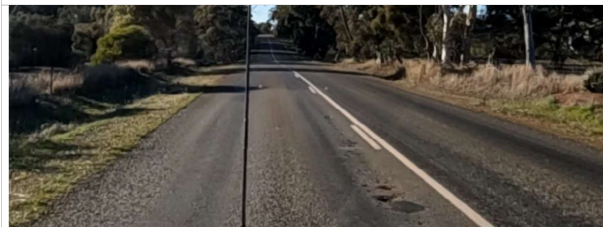
SLK 14.30 – Potholes forming (EB) and minor flushing (WB)
