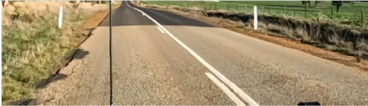
SLK 1.80 – Edge break and crack forming – Change of seal
