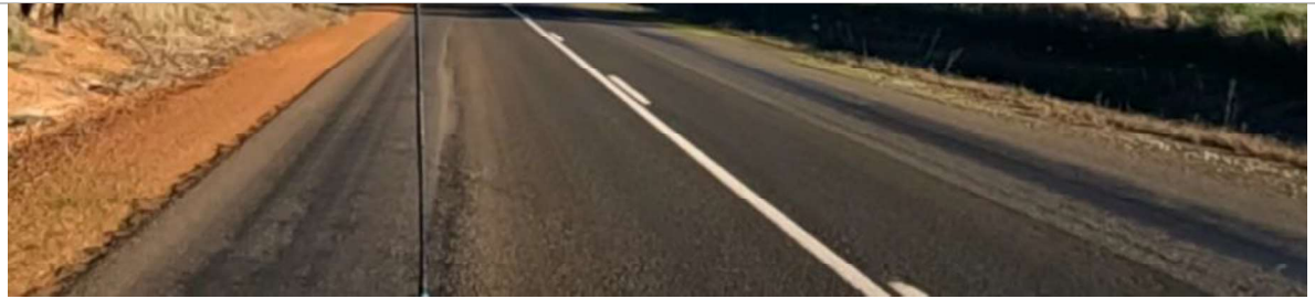
SLK 18.40 – Minor flushing (EB), crack and ravelling (WB)
