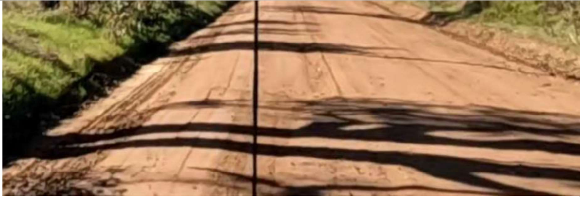
SLK 10.10 – Minor corrugation and rutting along the wheel path (EB)
