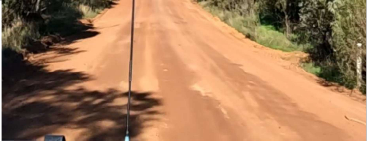
SLK 14.85 – Corrugation, minor rutting and base course exposure
