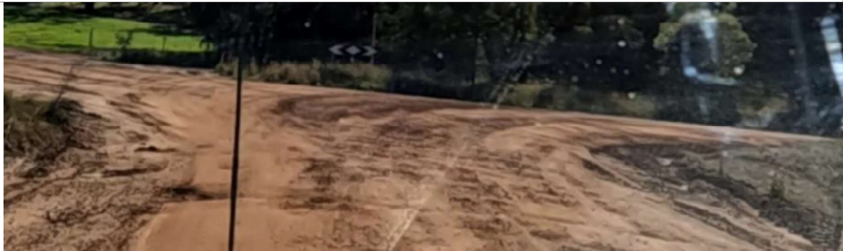
SLK 13.65 – Potholes and minor raveling approaching Yarranup Road
