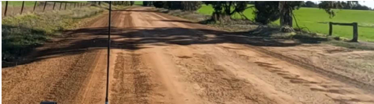
SLK 11.00 to SLK 11.20 – Severe corrugations and poor rideability with uneven surface
