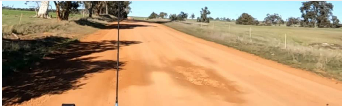
SLK 14.20 – Large potholes near culvert
