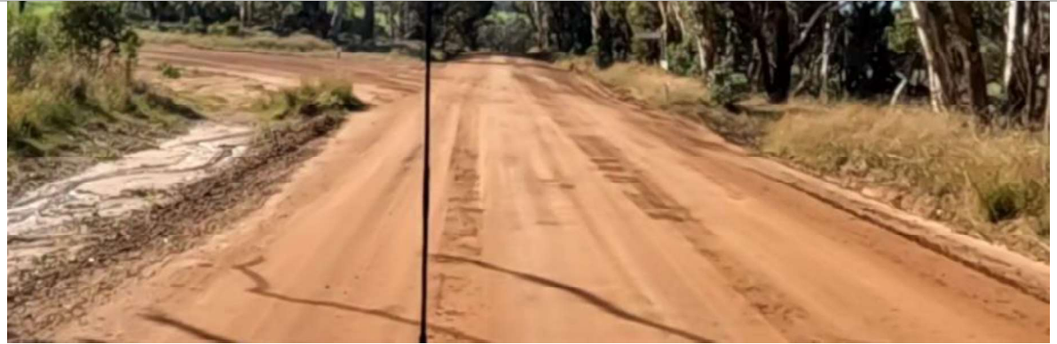
SLK 8.60 – Minor ravelling and potholes forming
