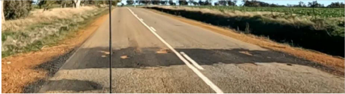
SLK 1.70 – Potholes forming on seal patch
