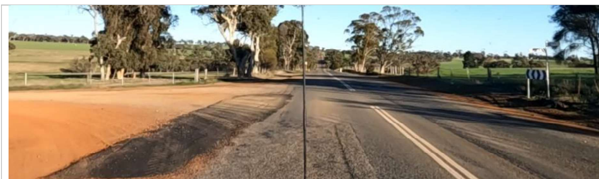
SLK 11.30 – Edge break and potholes forming at Bessen Road intersection
