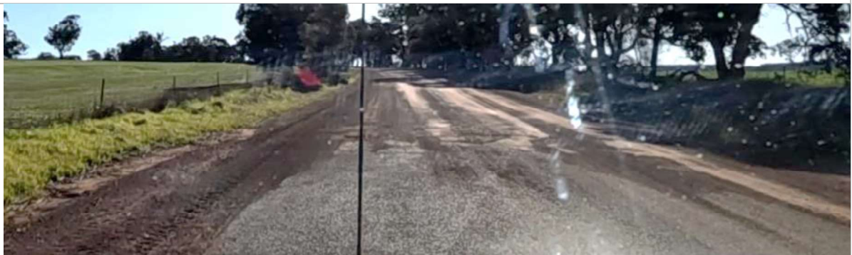
SLK 7.10 – End of sealed section. Ravelling and large pot holes near change of seal
