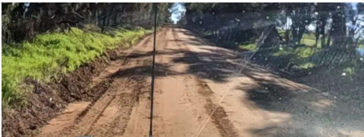
SLK 14.70 – Rutting, corrugations, uneven road surface with poor rideability
