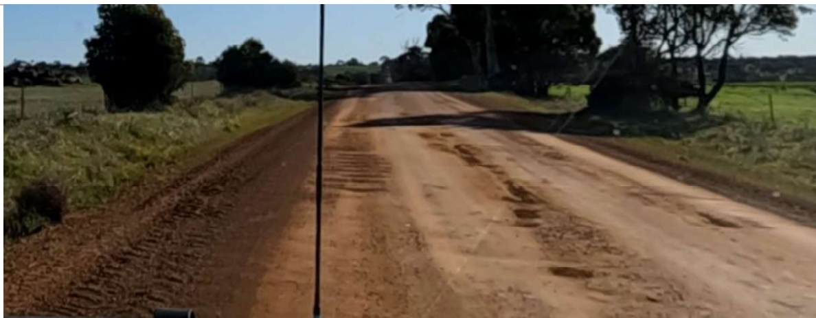
SLK 13.70 – Corrugation, raveling and potholes forming near the bend
