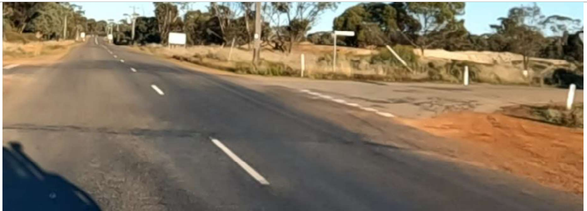
SLK 1.50 – Flushing near the intersection of Brown Street
