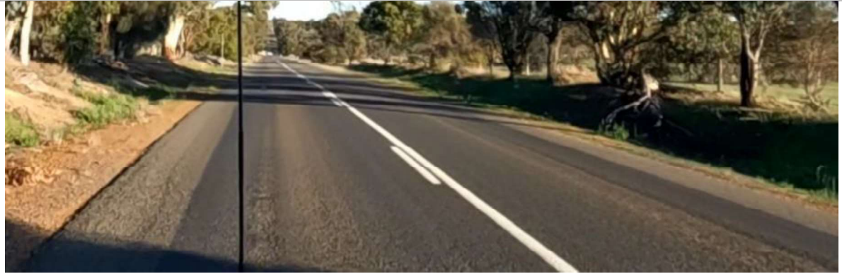
SLK 14.80 – Minor flushing
