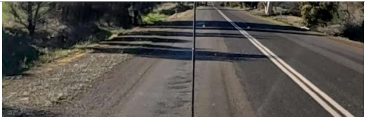
SLK 18.80 to SLK 18.90 – Minor flushing, minor ravelling with potholes forming
