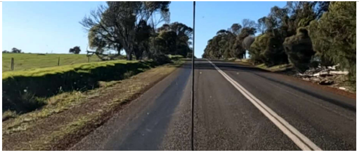
SLK20.00 – SLK 21.20 Minor flushing and minor ravelling along seal joint (EB)
