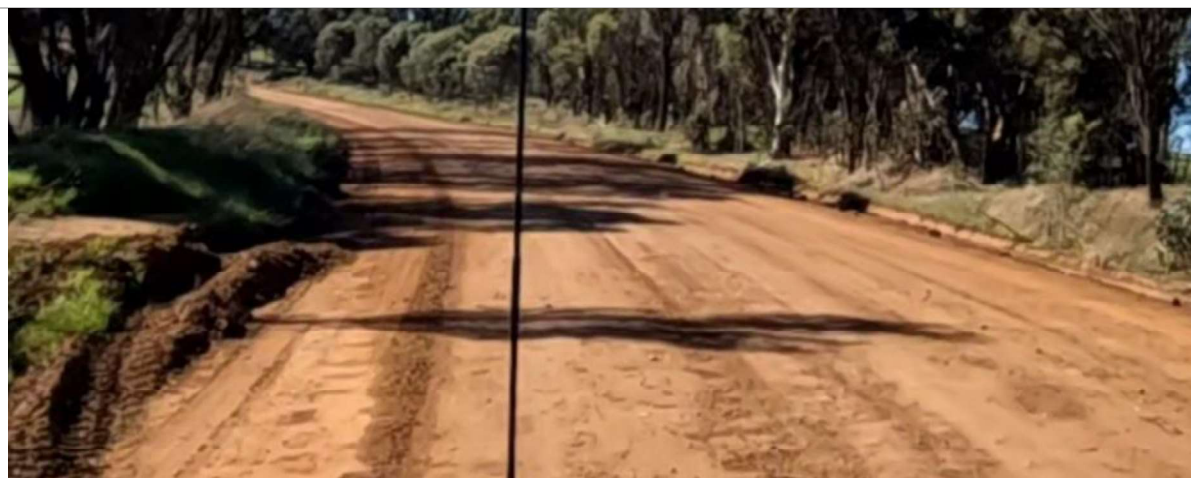
SLK 9.30 – Minor ravelling and corrugation along the wheel path along the bend
