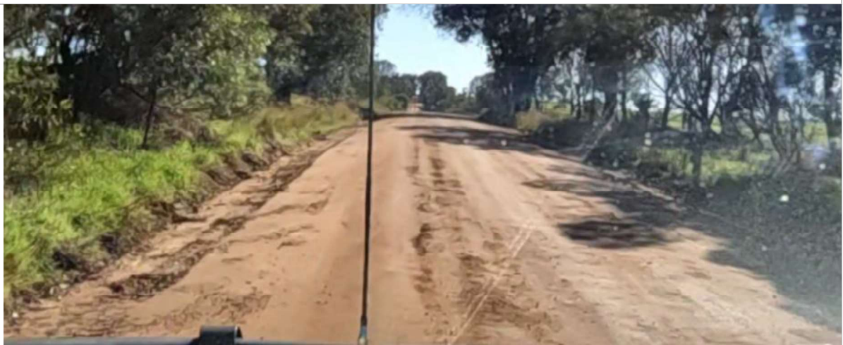
SLK 15.10 – Rutting, corrugation and potholes near farm crossover
