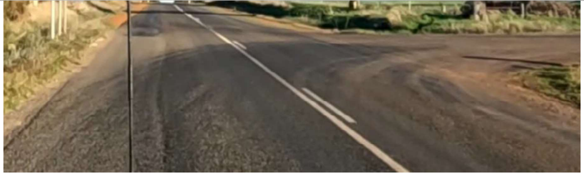
SLK 18.30 – Flushing and minor cracks forming near Birt Road Intersection
