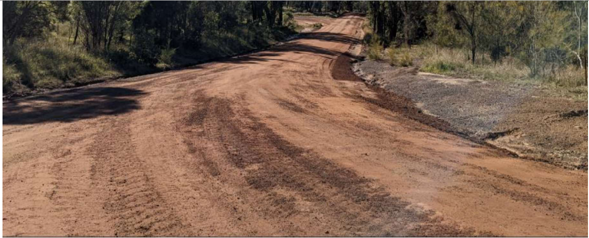
SLK 13.60 – Minor corrugations at the intersection of Yarranup Road
