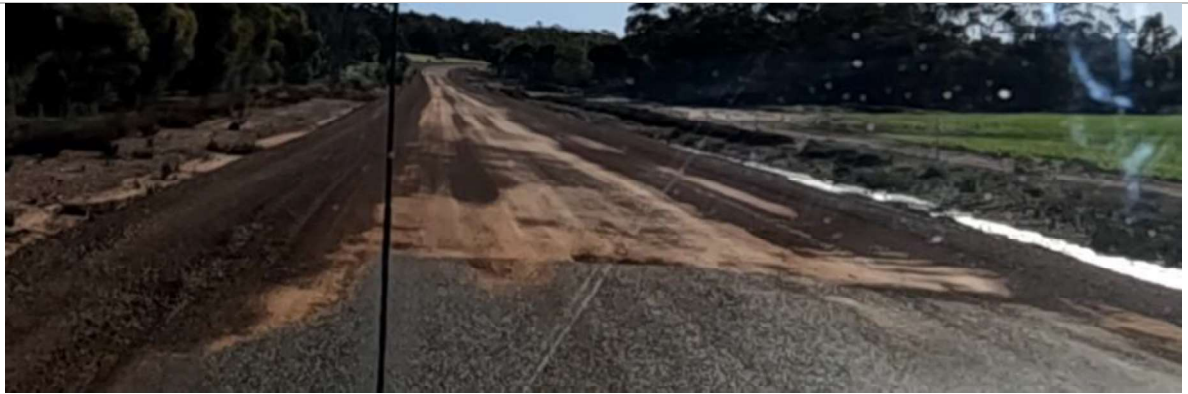
SLK 3.00 to 3.40 – Unsealed section, potentially washed out or damaged. Moderate corrugations
