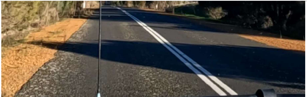
SLK 0.20 – Minor Edge break and minor ravelling
