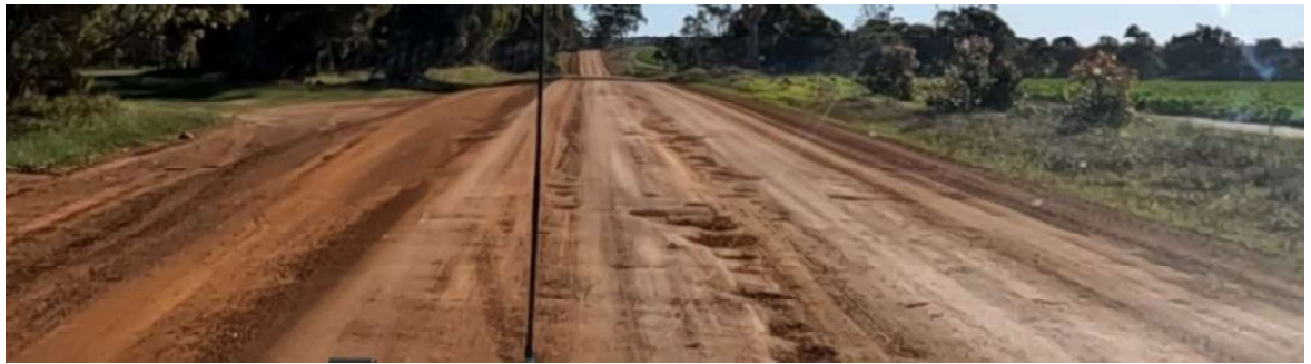
SLK 16.80 to SLK 17.00 – Severe potholes near Ngopitchup Road intersection
