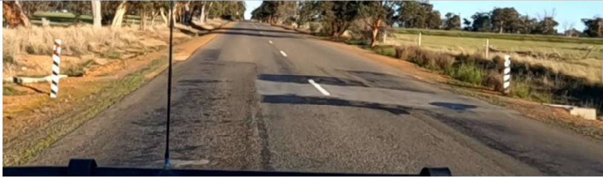
SLK 4.90 – Pavement seal patch failing with minor cracks
