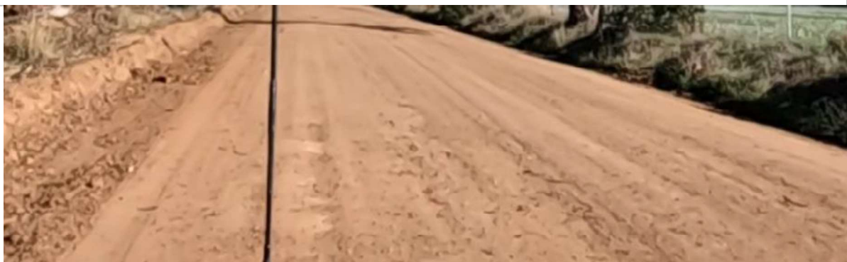
SLK 11.30 – Corrugation, rutting along wheel path
