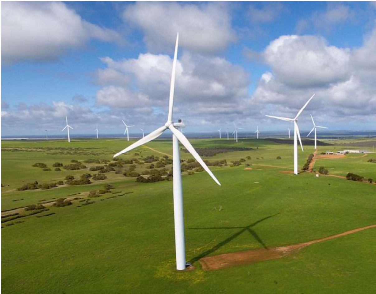
Plate 1: Typical turbine (photo courtesy of Western Power), a clear base within open land (pasture), retained crane pad and access track.
